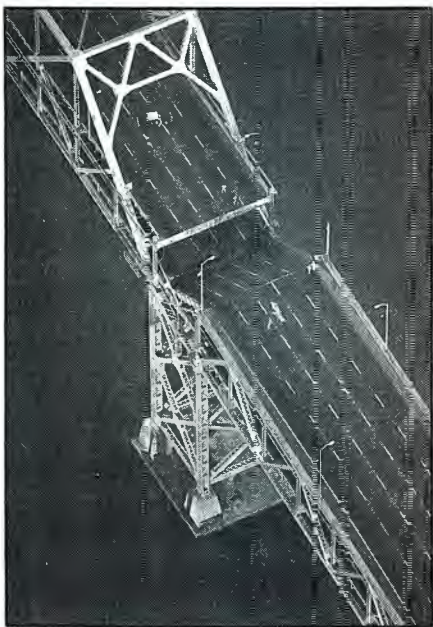
The importance of building high-rise and high-weight structures on bedrock was emphasized by the failure of a portion of the Bay Bridge, which runs between San Francisco and Oakland. The concrete pier moved during the quake, pulling the bridge apart like a toy. (Photo by Deanne Fitzmaurice, San Francisco Chronicle.)
