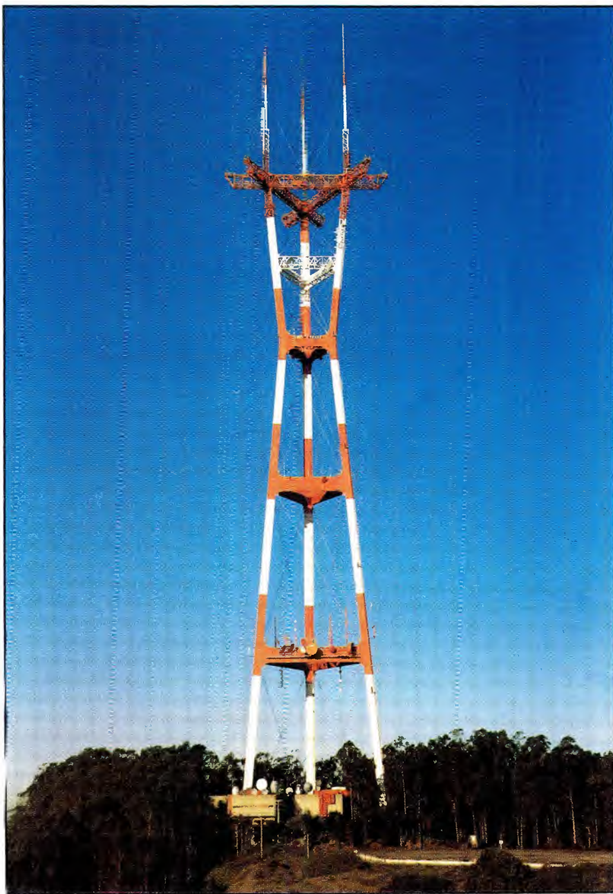
The shared transmission facility on Mount Sutro in the middle of San Francisco came through the earthquake in perfect shape. Built on bedrock, the 977-foot tower and its arrays are designed to withstand a quake measuring at least 8.3 on the Richter scale. During the quake, the tower moved, but stayed well within its design parameters. (Photo by Don Lincoln, Sutro Tower.)
